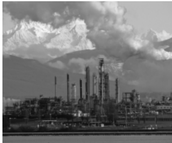
Oil Refinery in Anacortes, Washington
